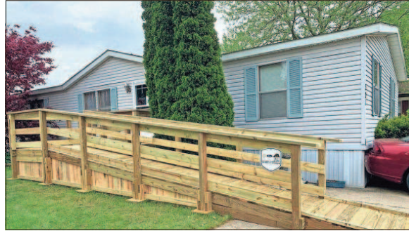
A ramp built by volunteers with Project Ramp. [COURTESY PHOTO]
